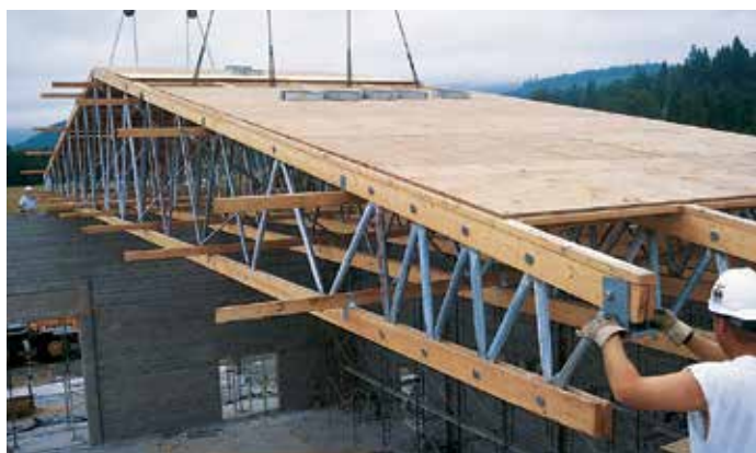
These heavy-duty, long-span pitched trusses are installed modularly. PHOTO CREDIT: RedBuilt
