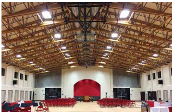
These scissor trusses help create multi-purpose space for Taylor Middle School. PHOTO CREDIT: RedBuilt
