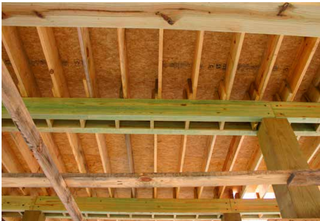
Shown during construction, treated glulam beams are set on piers to support the floor system above.
