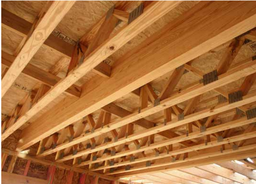
Glulam beams combined with trusses create an open, flexible floor plan.
