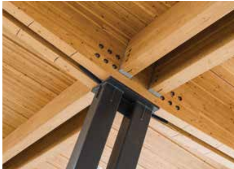
FIGURE 6 Concealed connections
