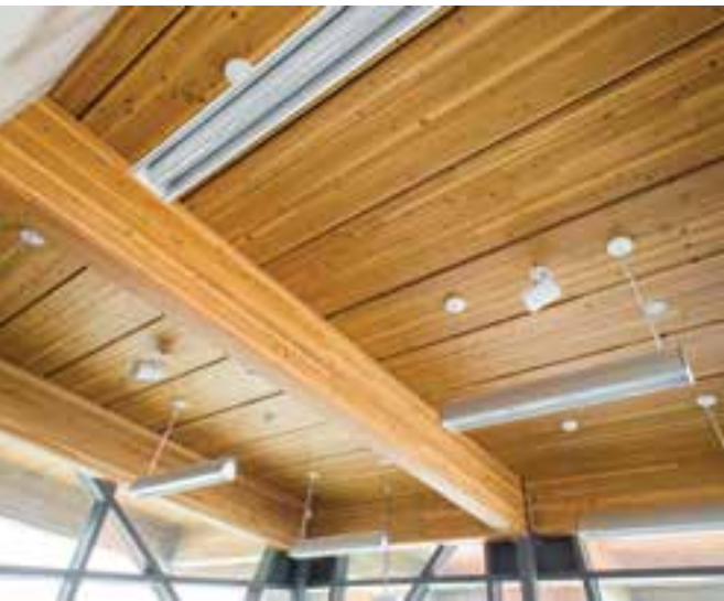
FIGURE 14 Bus Transit Station waiting room ceiling
