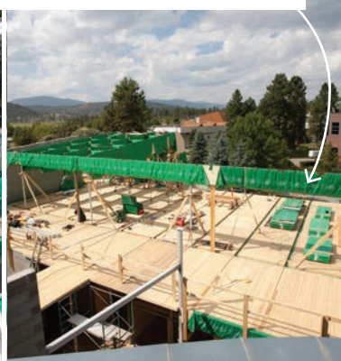
Roof Level: CLT Transfer Beam
