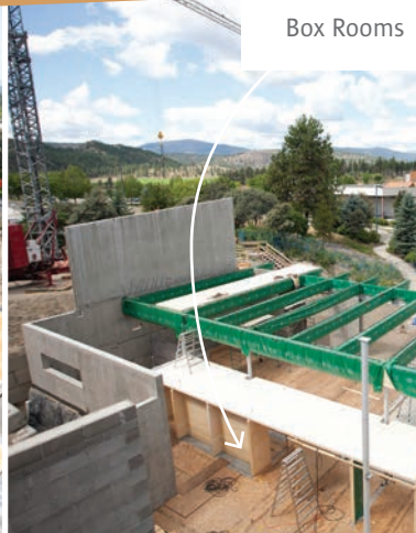
Roof Level: CLT Transfer Beam
