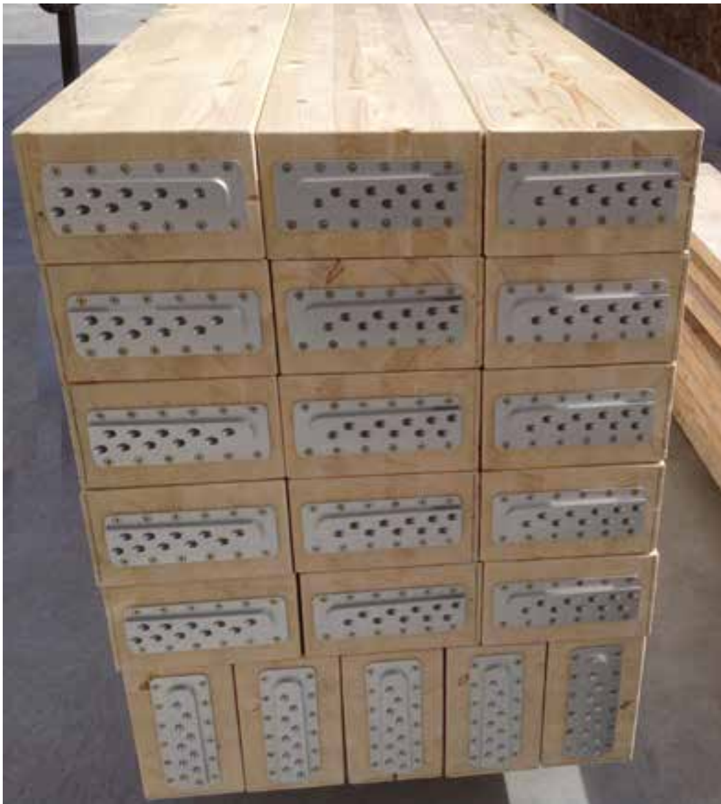
Modern timber connectors installed on wood. Photo credit: Herrmann's Timber Frame Homes
